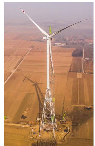
Truss Tower 170m
